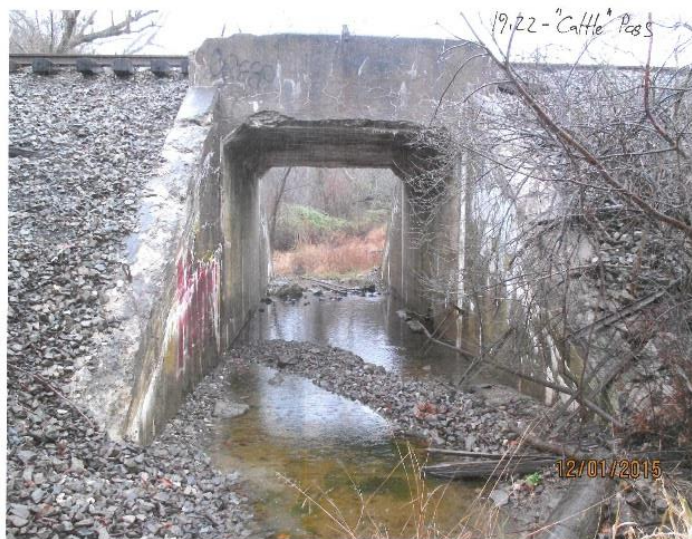
Figure 5-5 - Bridge 19.22 Cattle Pass
