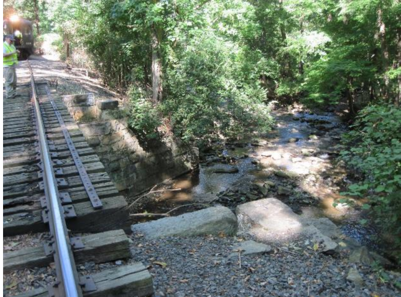
Figure 4-2 - Chester Creek at Structure 25.09
