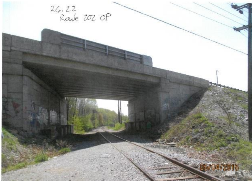
Figure 5-6 - Bridge 26.22 Overhead Bridge
